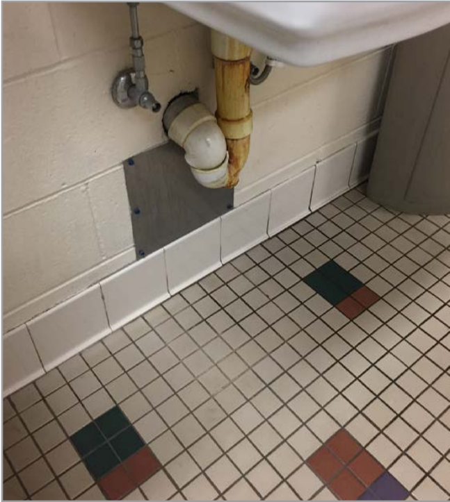
Replace pipe covers in the Toilet Rooms
