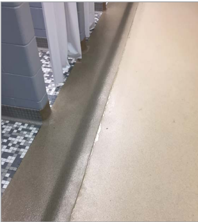
Replace epoxy floor in Girls Varsity Locker Room C140
