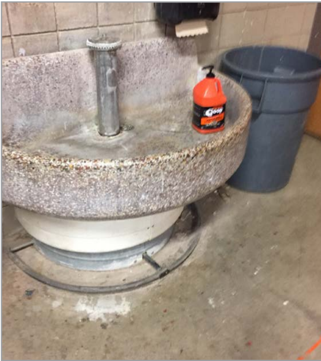
Replace wash fountain in Tech Ed C100
