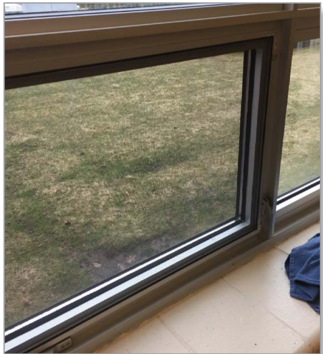
Replace leaking window
