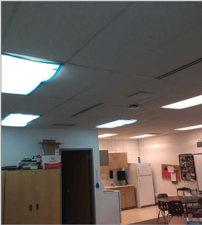
Provide new light fixtures in Special Ed A104
