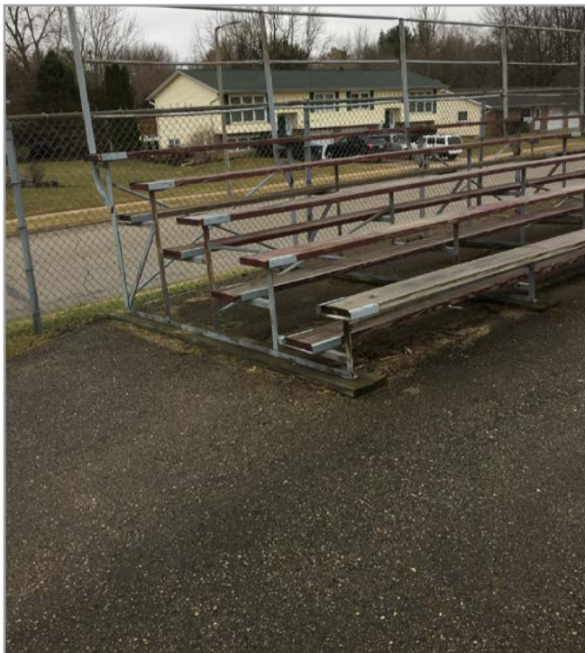
Replace unsafe visitor football bleachers
