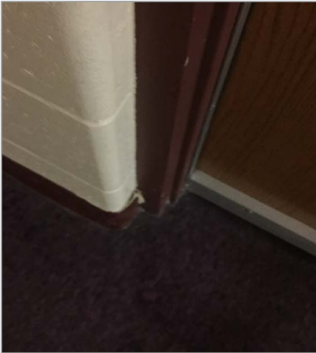
Provide premolded corner floor base
