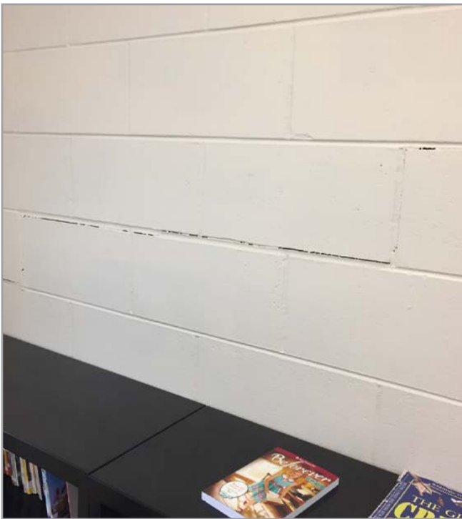
Repair mortar joints in masonry wall
