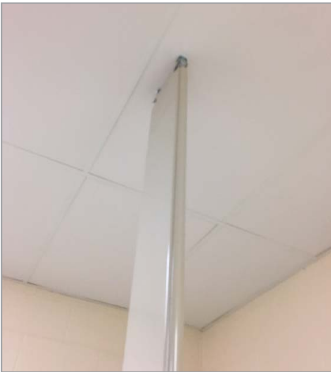
Replace toilet partitions with floor mounted overhead braced partitions
