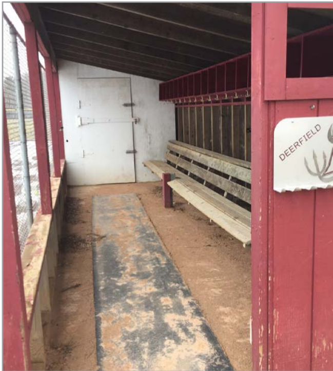
Replace existing Softball dugouts
