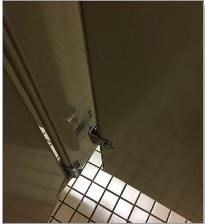
Replace damaged toilet partitions
