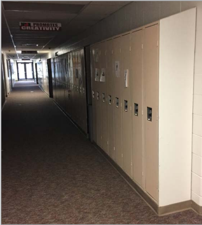
Upgrade floor finish to epoxy in Corridors
