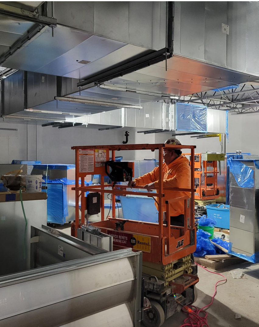
AIR HANDLERS BEING INSTALLED
