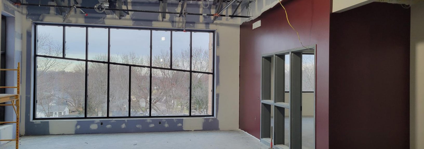
GLASS INSTALLED ON SECOND FLOOR
