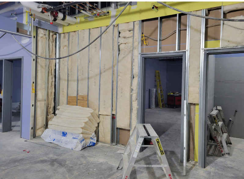
INTERIOR INSULATION BEING INSTALLED
