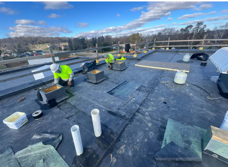
DETAILING ROOF PENETRATIONS
