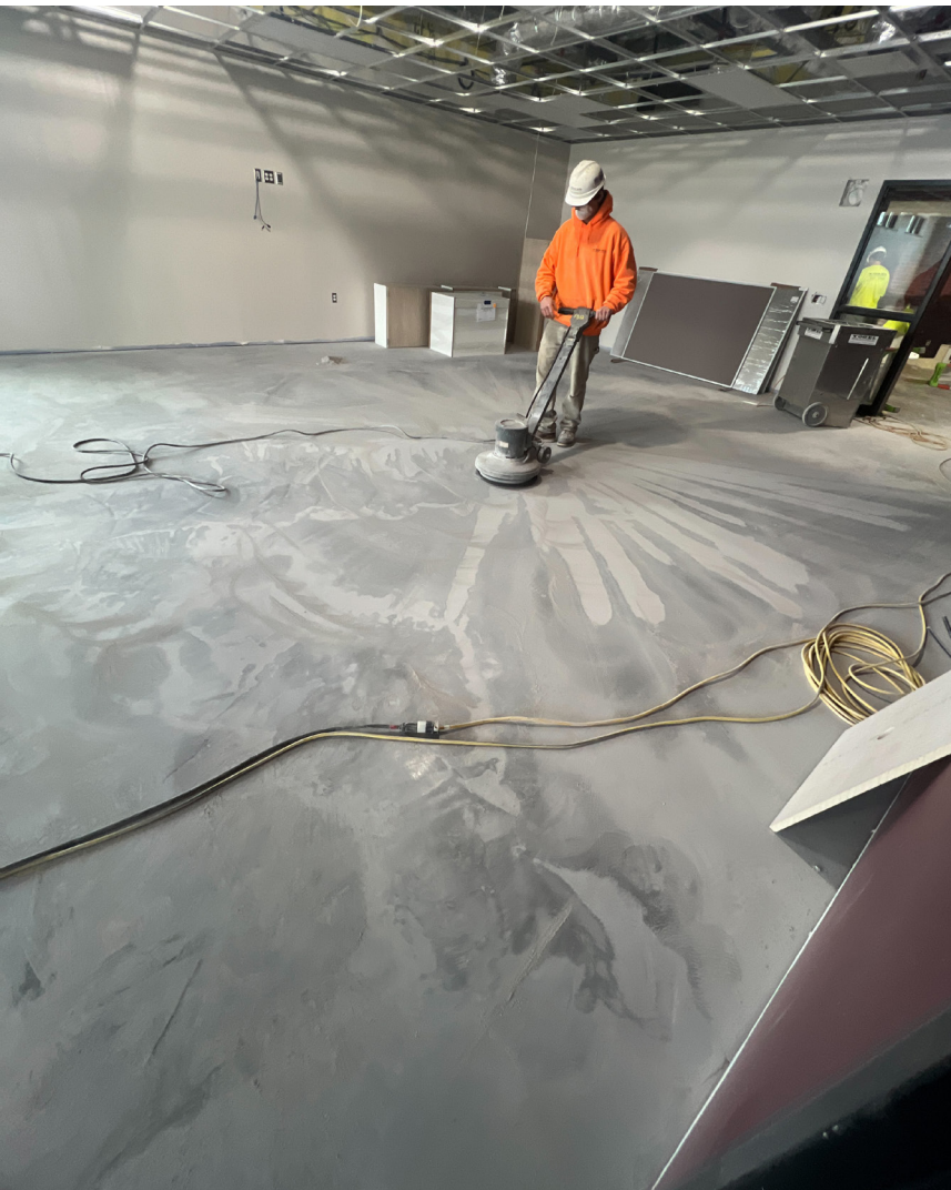
CONCRETE BEING SANDED FOR FINISH FLOORING
