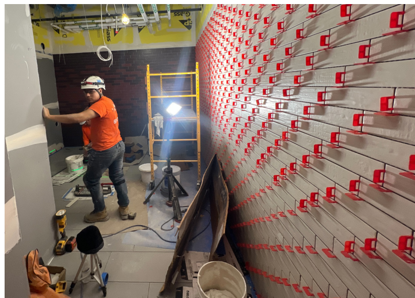
INSTALLING BATHROOM TILE
